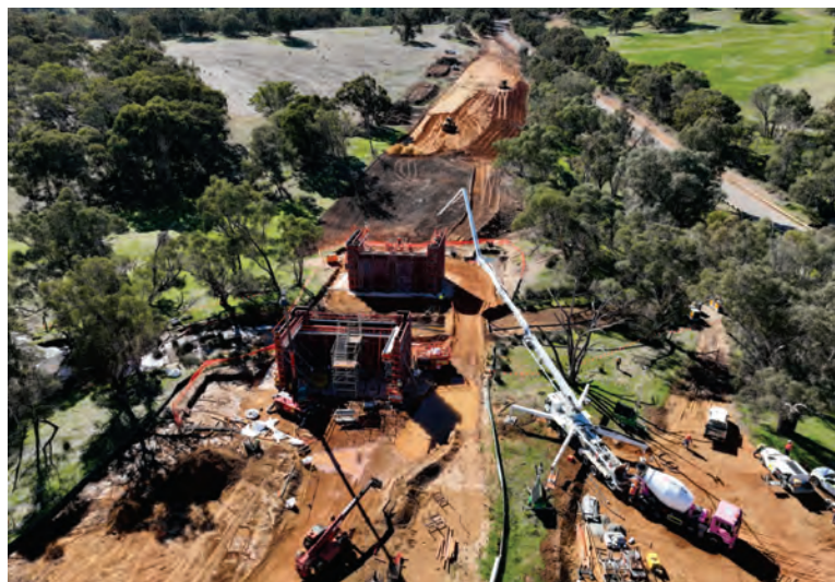
Construction work in full swing at the Jimperding Brook bridge site
