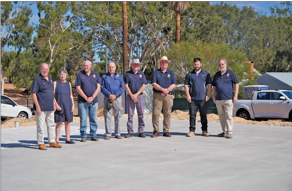
The initial concrete pour for the Toodyay RSL's new home marks a major milestone.
