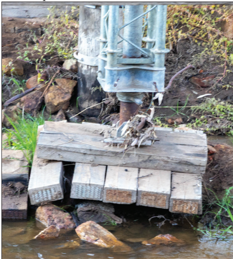
Slaughterhouse Bridge support undercut by water erosion. (May 2025).
