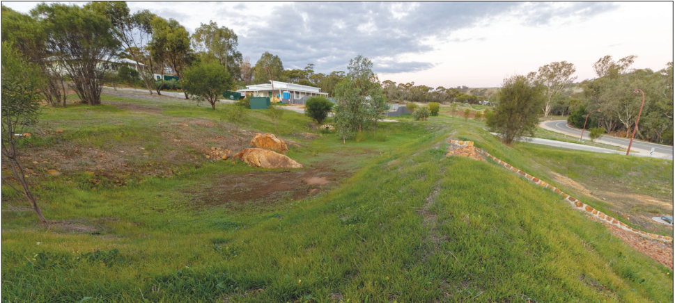
Drainage sump at the corner of Rayner Loop and Drummond Street East. The sump is on two levels and used to contain waterflow from Rayner Loop. This patch of shire-owned land is intended to be rezoned to public open space.
