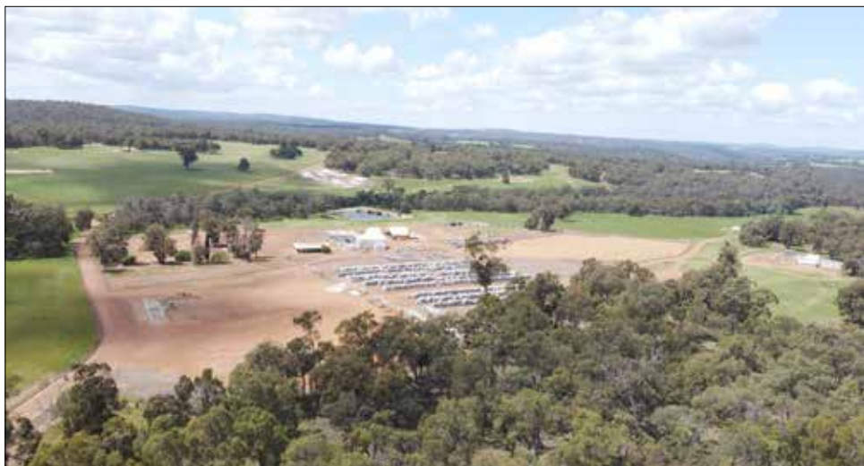
Chalice Mining’s worksite at Keating Road, Julimar, where the Gonnevillie Project is planned to be a critical minerals mine approximately 70km north-east of Perth.
