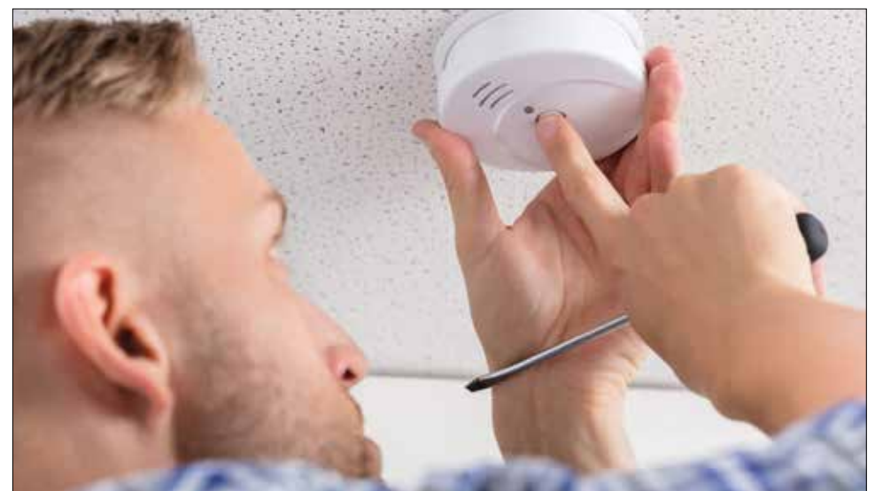
Checking smoke detector.
