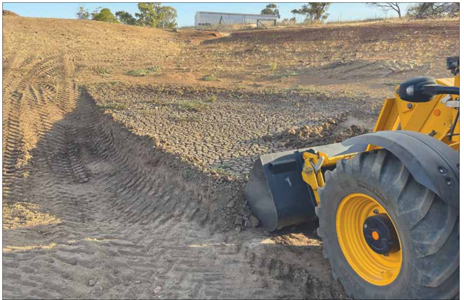
Local dam being cleaned of dry mud. Photo: Stephen Cook.
