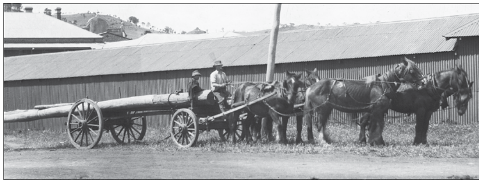
Team of horses hauling power poles into position. (Photo: Courtesy, Toodyay Shire Museums, 2008.52).
