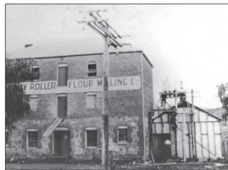
Power House shed next to the Mill. (Photo: Courtesy, Toodyay Shire Museums, 2012.30).
