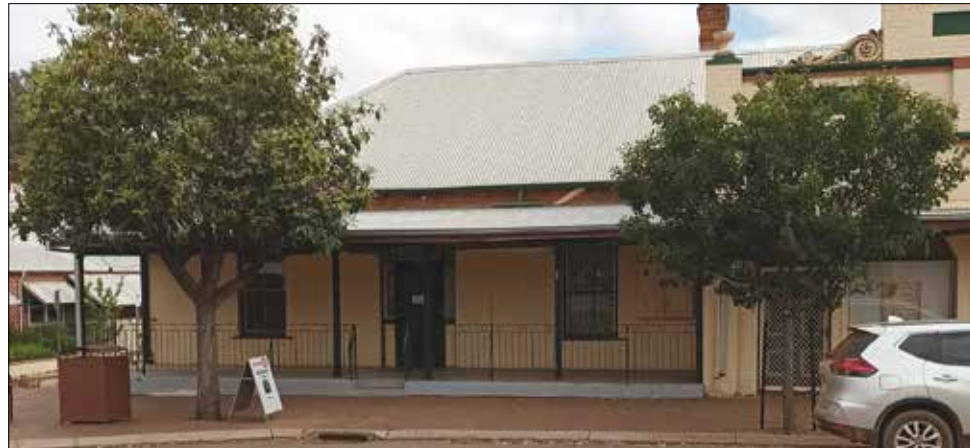
The St John Sub Centre Administration building on Stirling Terrace before the painting upgrade.
