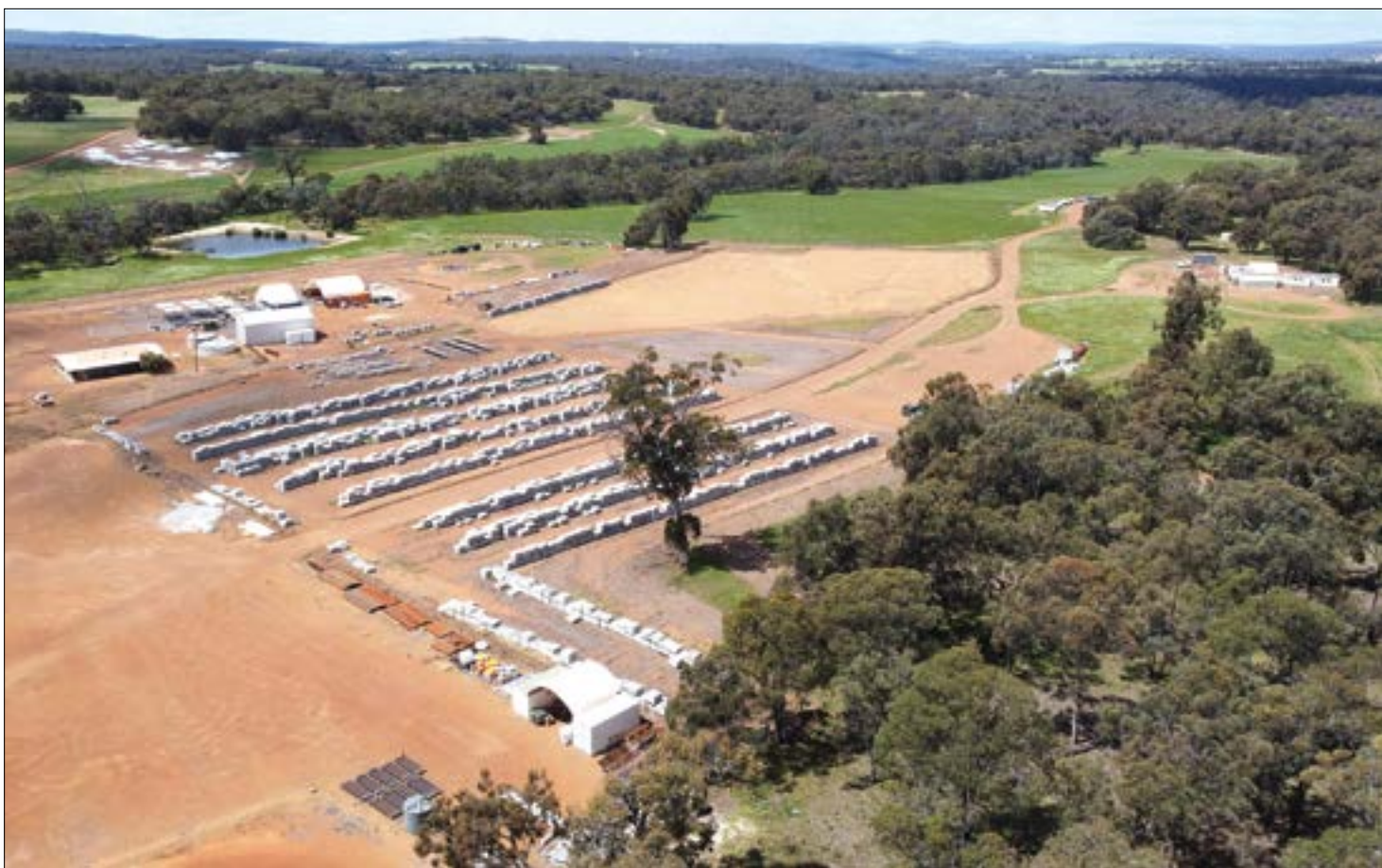
Chalice Mining's worksite at 229 Keating Road where the company has announced plans to create a massive open-cut mine measuring nearly two kilometres across, 1.5km wide and more than half a kilometre deep on a scale similar the world-famous Kalgoorlie Superpit.
