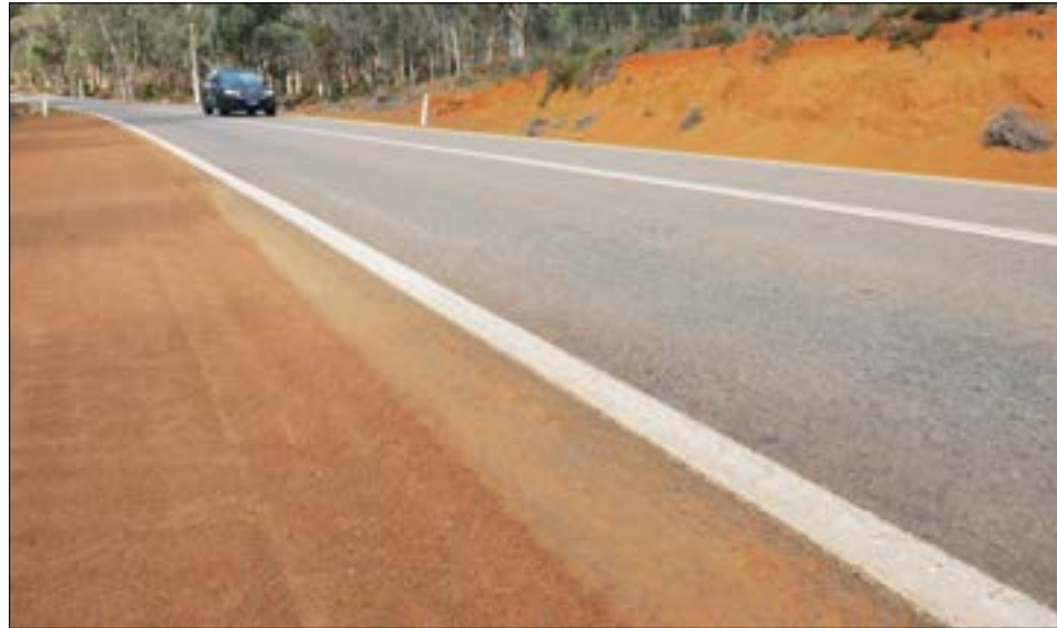
Recently repaired road edges on Toodyay Road.
