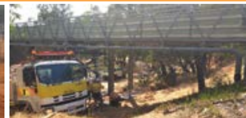
Newcastle Park Footbridge: Maintenance Repairs
