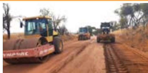
Bindi Bindi-Toodyay Rd: Regional Rd Safety Works
