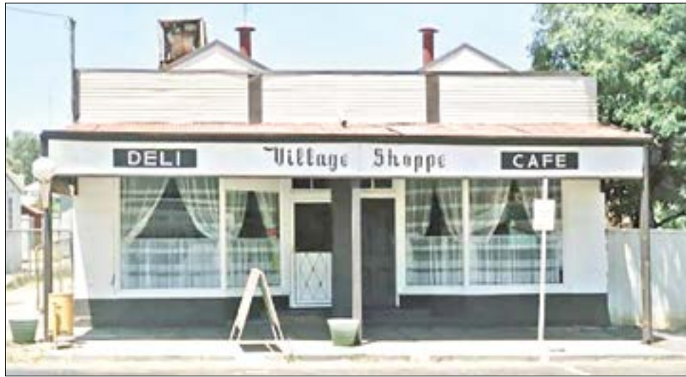
This former Stirling Terrace wine saloon in became a grocery store and then a real estate agency before it was destroyed by fire in 2009. Photo: WA State Library.
