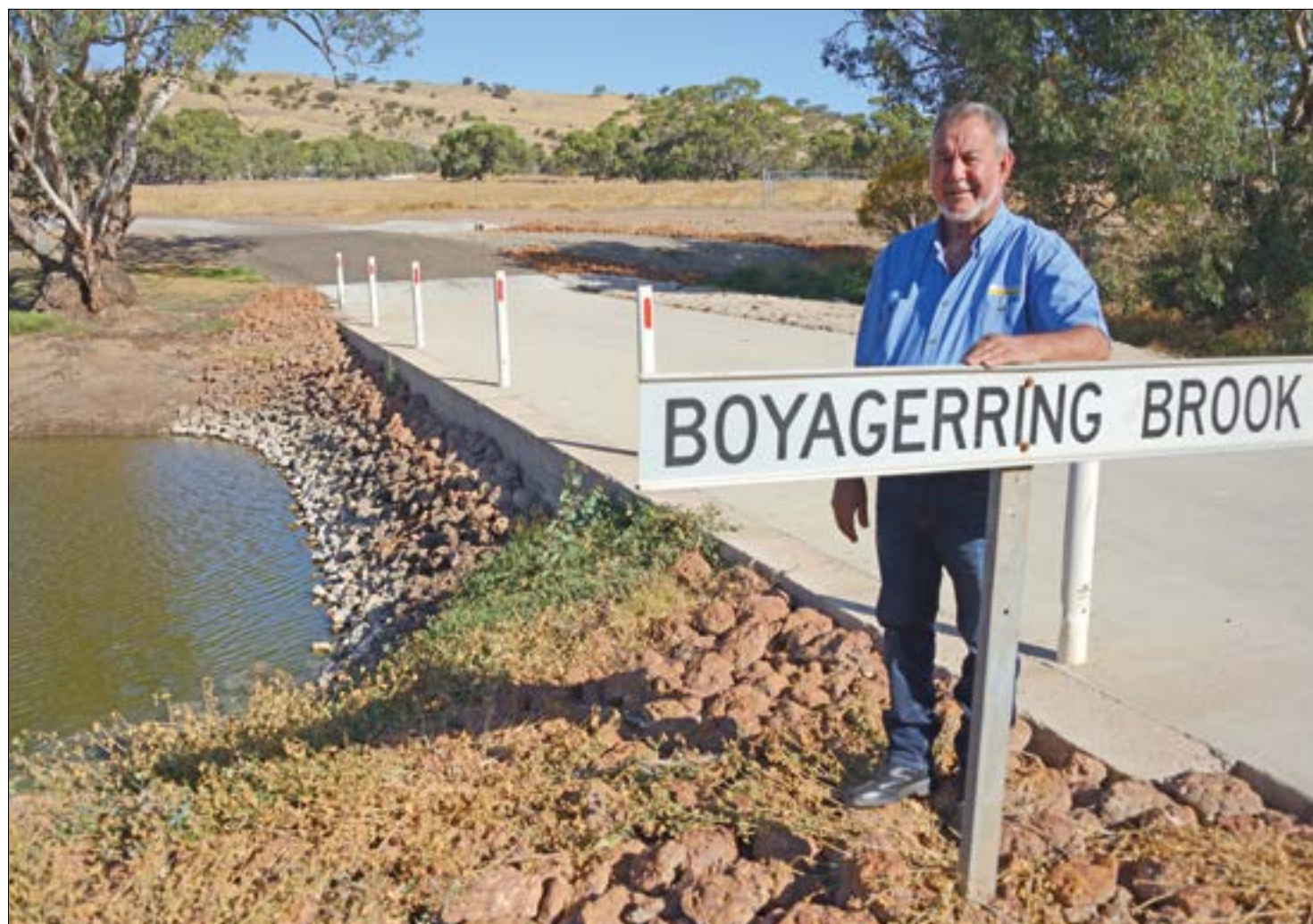
Local real estate agent Tony Maddox at the driveway, culvert and pond which threatens his livelihood and seven staff members' jobs.
