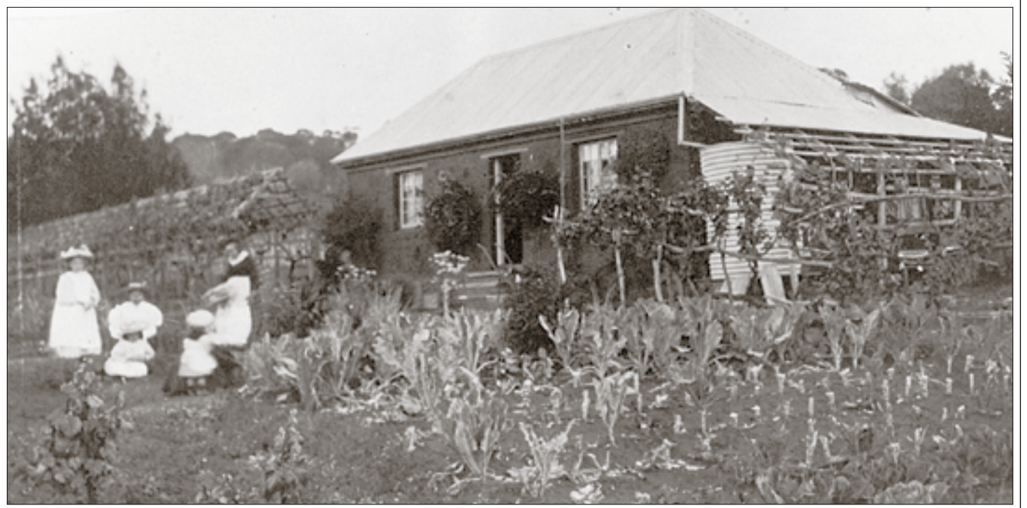
The way we were – this undated photograph shows an early 1870s workman's cottage in Folewood Road. The single-story brick and iron cottage with timber casement windows was built by Samuel Haggard and W Stevens and is regarded as an example of local Victorian architectural style and for its association with early settlers of the Toodyay district. Photo: Newcastle Gaol Museum.
