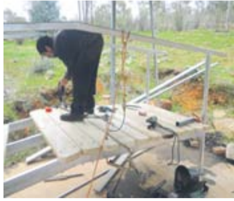
Constructing the footbridge for the Bilya Walk Track
